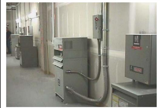
Multiple harmonic-suppressed transformers were used to power the building reliably without permitting harmonic current flow.
